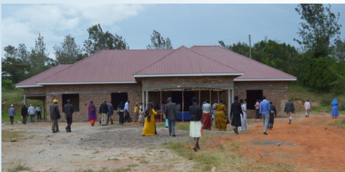
Front View of RACOB AO's new progress of RACOB AO's
